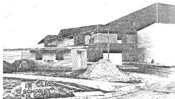
Phillip College under construction
